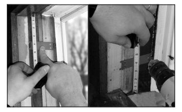
Note: Additional clips are supplied and may be used if required on taller units. Place the additional clips approximately at the midpoint of each sash location if necessary.
