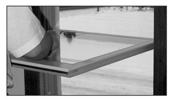
11. Tilt the sash upward until the tilt latches engage in the jambliner. Allow sash to drop and engage clutch mechanism. Repeat procedures 7 through 9 to install lower sash (using inside track). Both sash should fit snug against the jambliner.
