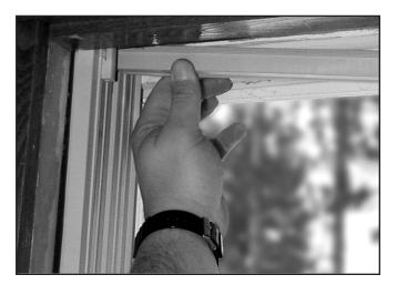
**9.** When installing the top sash, engage pin in the outside track of the left balance (tilt pin must be above clutch mechanism) then engage the pin in the outside track of the right balance (above clutch mechanism).
