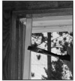
4. Verify the correct fit of the jambliners by placing them against the side jambs. If too tall, cut the bottom of the jambliners in 1/16" increments at a 14° angle. The supplied head jamb gaskets need to be applied to head jamb. Only two are needed - color match to jambliner. Peel off protective backing to expose adhesive and apply gasket to existing head jamb.
