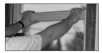
12. If applicable, replace the inside stops loosely against balance so that the balance can move freely. If the jambliner is not fully covered by the stops, additional stop material may need to be applied.
